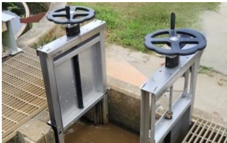
Image 56. Sluice gates
